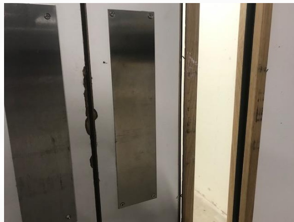
Example of 6 month old doors below due to damage of bins taken in and out.
